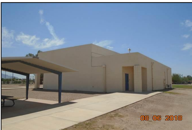
Picture 11 - Picture 10 – Concrete block and mortar exterior walls with white paint found on the Gymnasium
