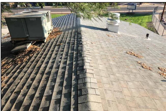
Picture 5 – Asphalt shingles and felt roofing system found on Buildings 5 through 14.
