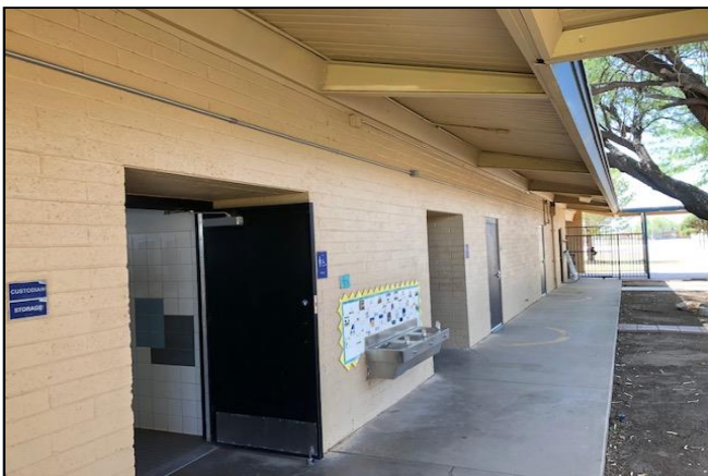
Picture 9 – Concrete block and mortar exterior walls on buildings 5 though 14.
