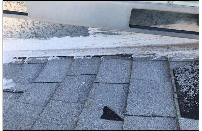
Picture 8 – White roof sealant on HVAC systems on buildings 5 through 14 and the Gymnasium.
