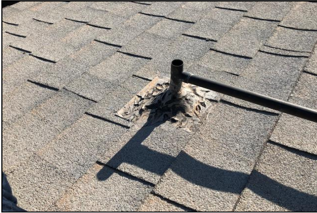
Picture 7 – Black roof penetration sealant found on buildings 5 though 14 and the Gymnasium.
